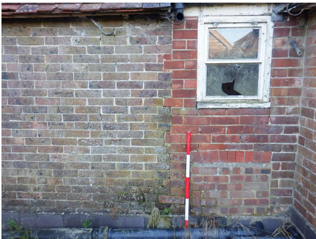
Plate 5. North façade replacement window (see Plate 2-red arrow)
