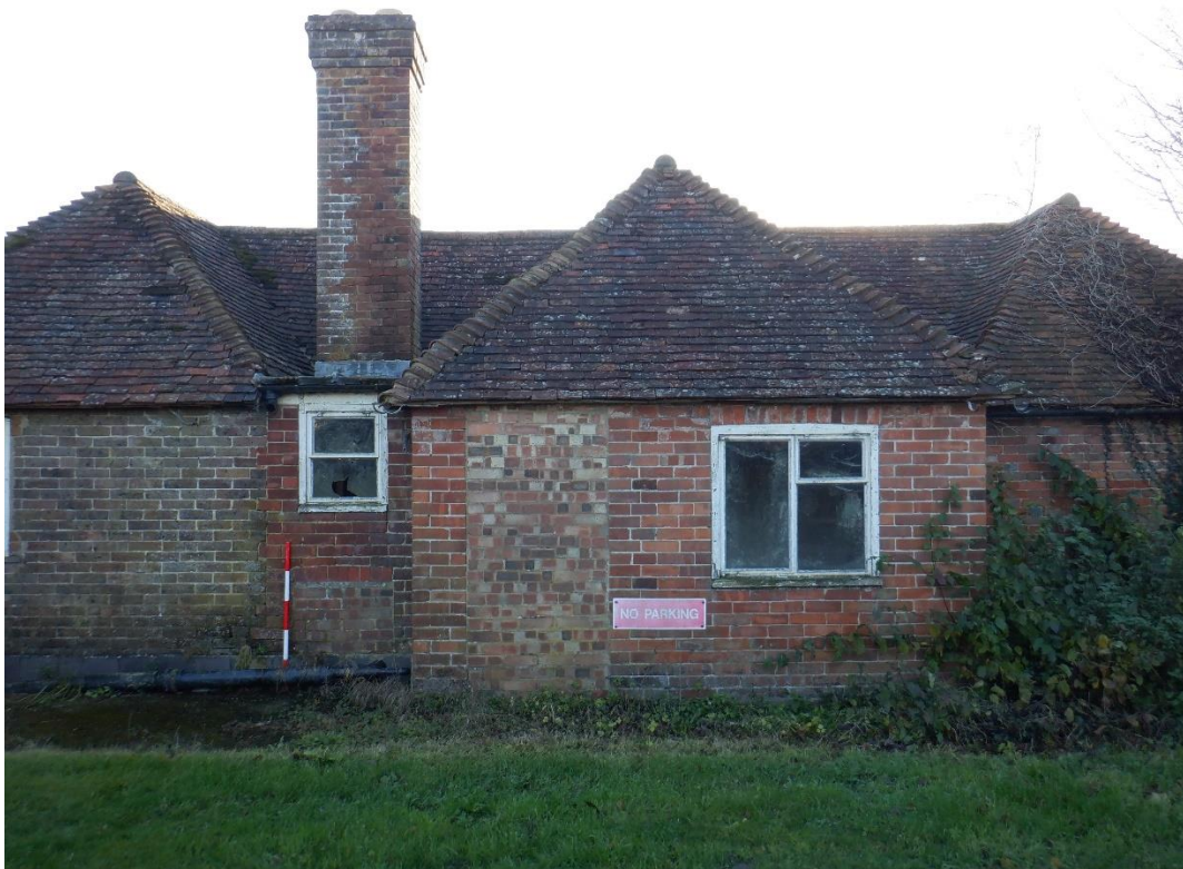
Plate 2. North façade (looking South) Note blocked up doorway- red arrow (1m scale)
